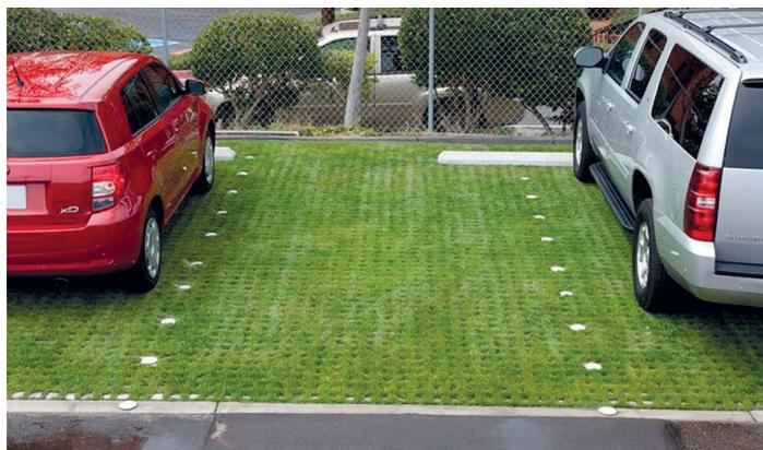
Here the plastic grid is filled with topsoil and seeded with grass. This system can be used on the access road, as well as for an overflow parking area
