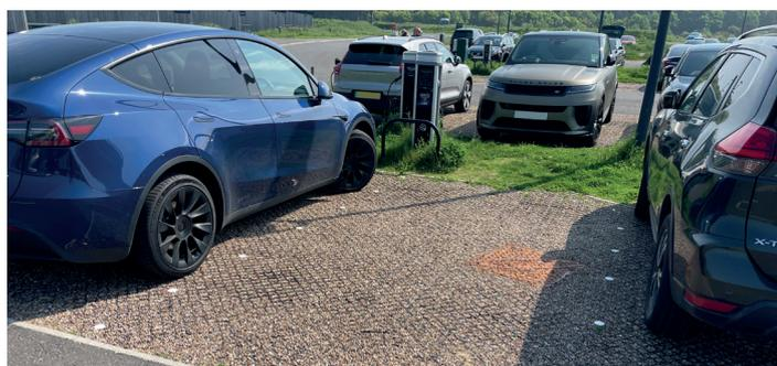
Car parking space composed of a plastic grid, filled with fine gravel, which is laid over a road-stone base. Also note – the electric car charging station
