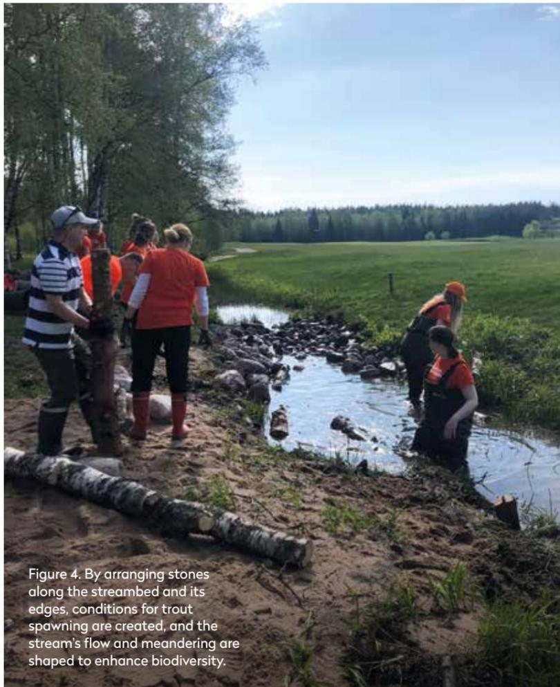
Figure 4. By arranging stones along the streambed and its edges, conditions for trout spawning are created, and the stream's flow and meandering are shaped to enhance biodiversity.
