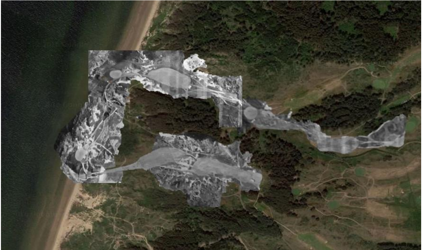
Figure 2.6 Aerial photography from 2020 overlain by historical aerial photography from the 1960s to show the extent of erosion at the Formby course
