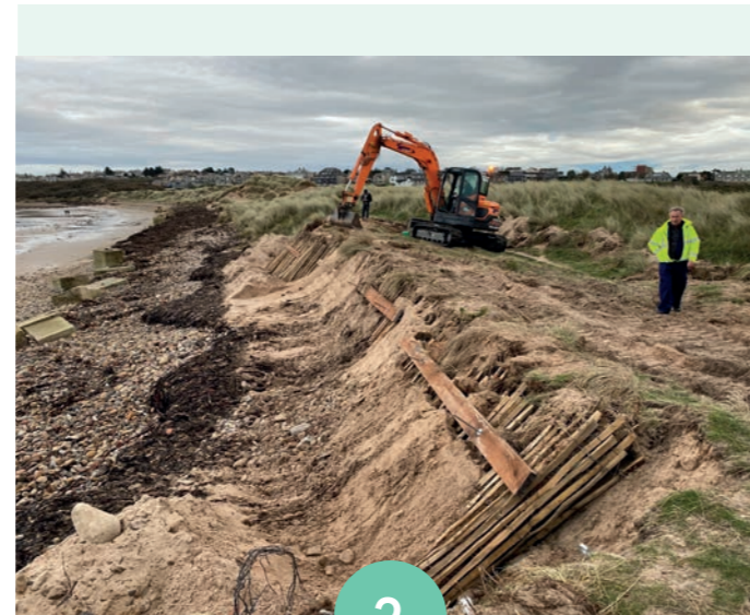
Re-grading of sand cliff
