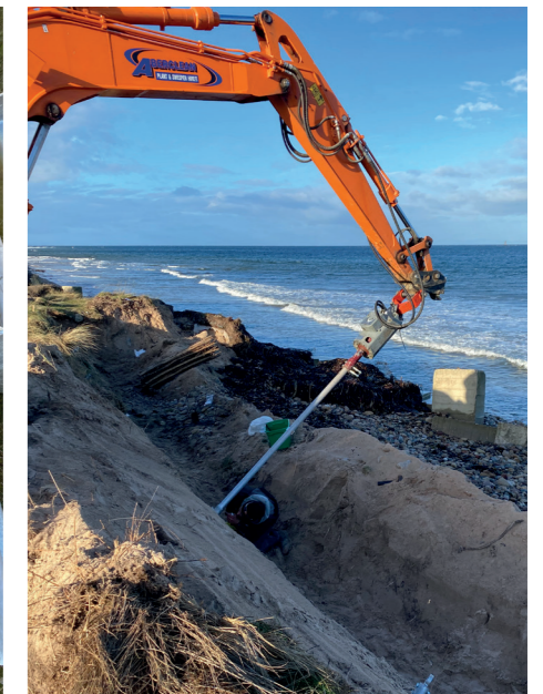
Fig B. Screw pile installation at Moray GC
